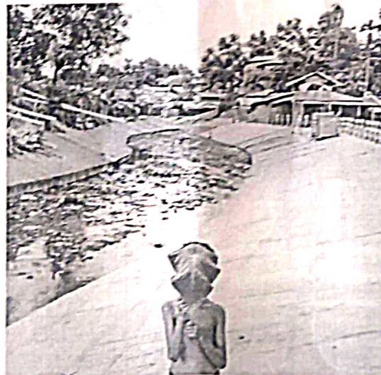
Figure 2: The open drain that now runs through the crowded centre of Kutupalong camp
