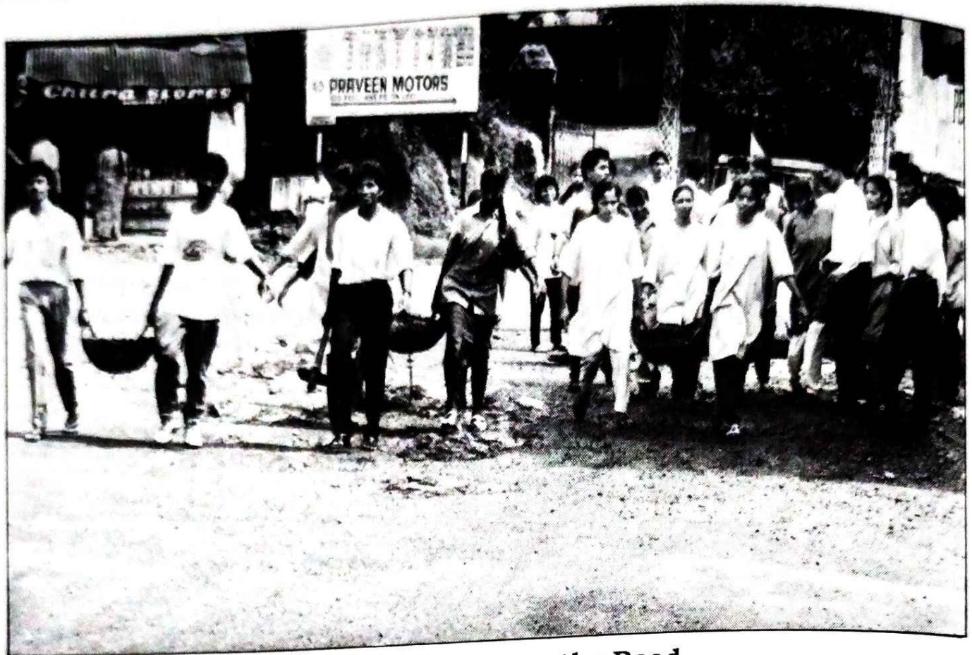
Students Repairing the Road.
